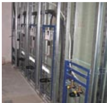
Example: Installation in partition walls in domestic areas with HERZ pipes
