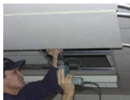
Installation of cooling ceiling
