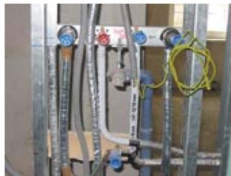
Example: Installation in partition walls in domestic areas with HERZ pipes
