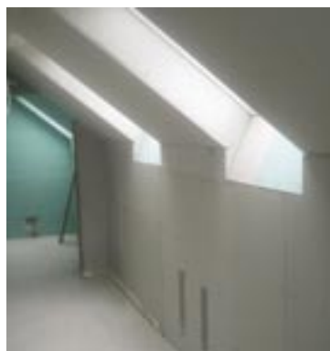
Renovation of apartments
